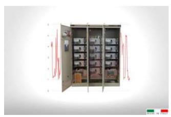
The AAR/6 series are suitable for three-phase networks with an operating voltage of 400 Vac and very high harmonic current content with values that do not comply with EN50160 (wire drawing, chemical-pharmaceutical or oil industries. Heavy Duty capacitors with double elements and increased thickness allow use even in extremely harsh working conditions
