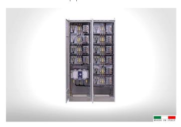
The entire **AAR/100-ST** series is equipped with "zero-crossing" static relays (thyristors), and it has been designed to improve the performance of traditional equipment, such as: increasing the life of the capacitors banks, decreasing the time response of the equipment to follow rapid changes in loads. Suitable for applications with **high harmonic distortion** such as automotive, harbours, mechanical workshops, ...
