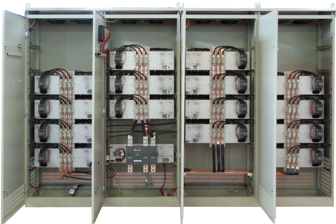
Photos of AAR / D20 1150 kvar installed
